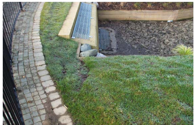
Figure 14.20: Swales at Upton, Northhampton, UK
