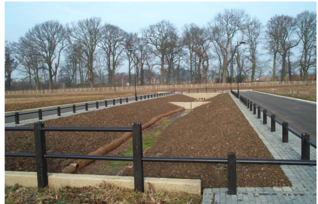
Figure 14.18: Swales at Upton, Northhampton, UK
