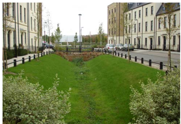
Figure 14.19: Swales at Upton, Northhampton, UK
